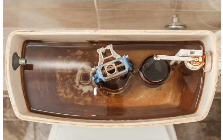
Iron bacteria in toilet tank
